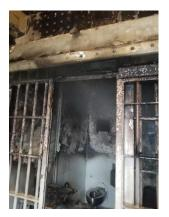
Puzzled, Mr. Antonetti contacted the Department to "determine why the heavy damage occurred with sprinkler protection in place. DOC indicated that the sprinklers protection for this area had been shut down due to a sprinkler being damaged by an inmate. The sprinkler was not replaced in a
